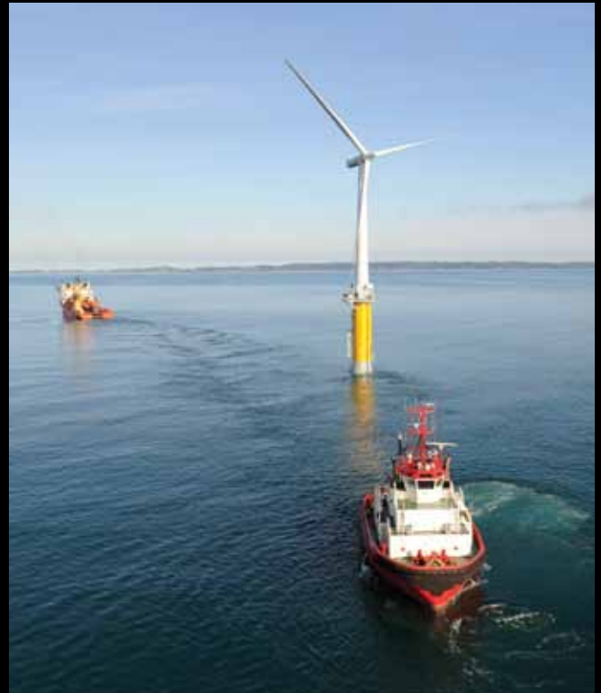
Technip installed the world's first full scale offshore floating wind turbine "Hywind"
