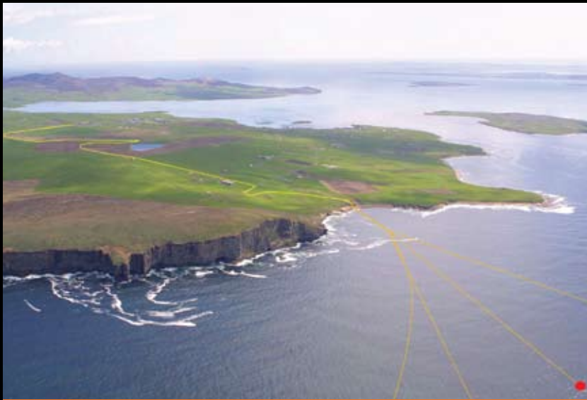
EMEC's Billia Croo wave energy site in Orkney: Yellow lines show where 11kV subsea cables lie descending to 50m depth, 1.2km from shore at locations 0.5km apart.
